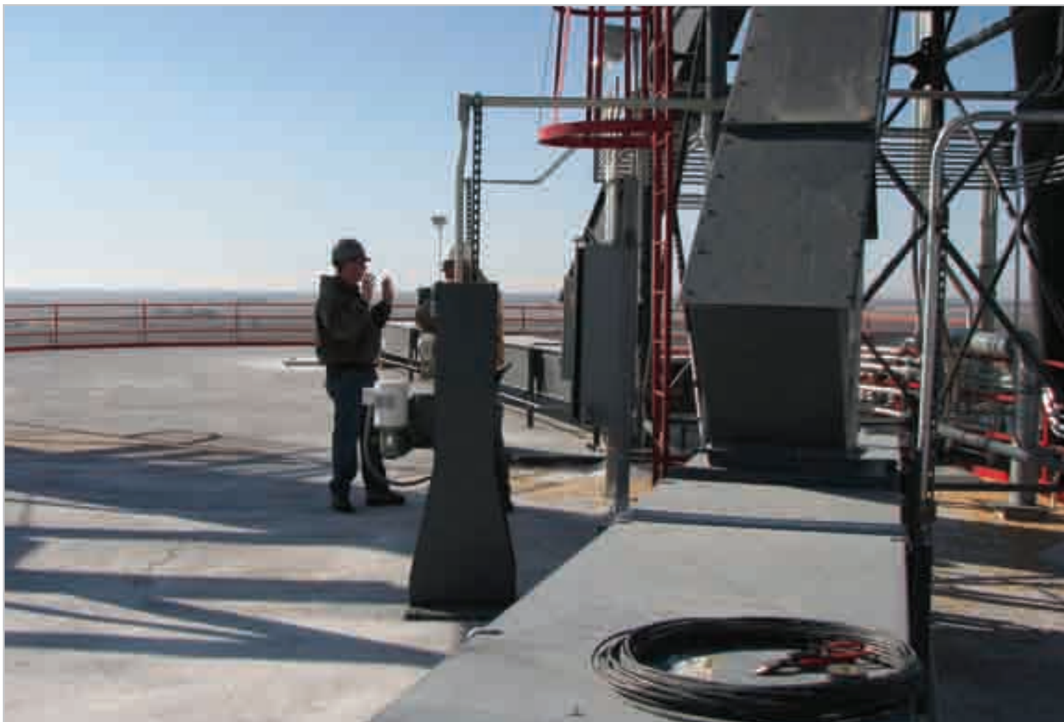
Conveyor fill on top of the silo.
