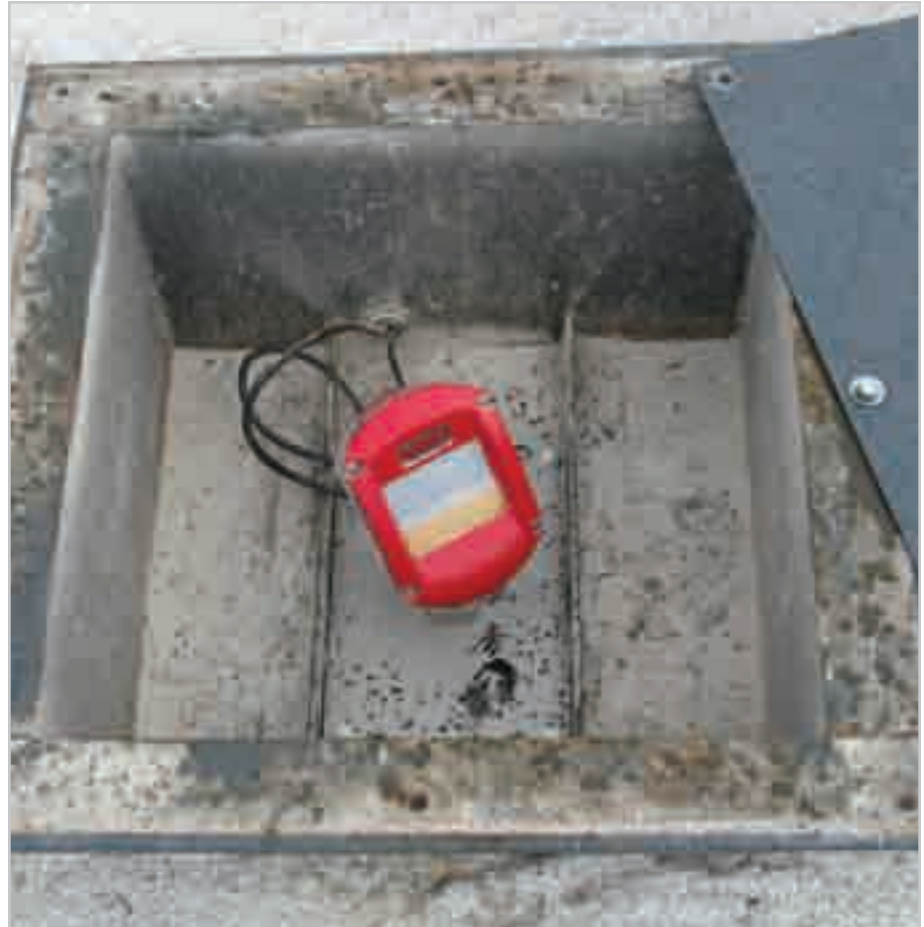
3DLevelScanner mounted on top of cement silo.
