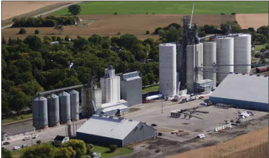
A new 450,000-bushel jumpform concrete silo built at Glacial Plains Cooperative at Murdock, MN in 2011 is visible at the far right. Aerial photo taken by R. DuMont/New Horizons Aerial Photography.
