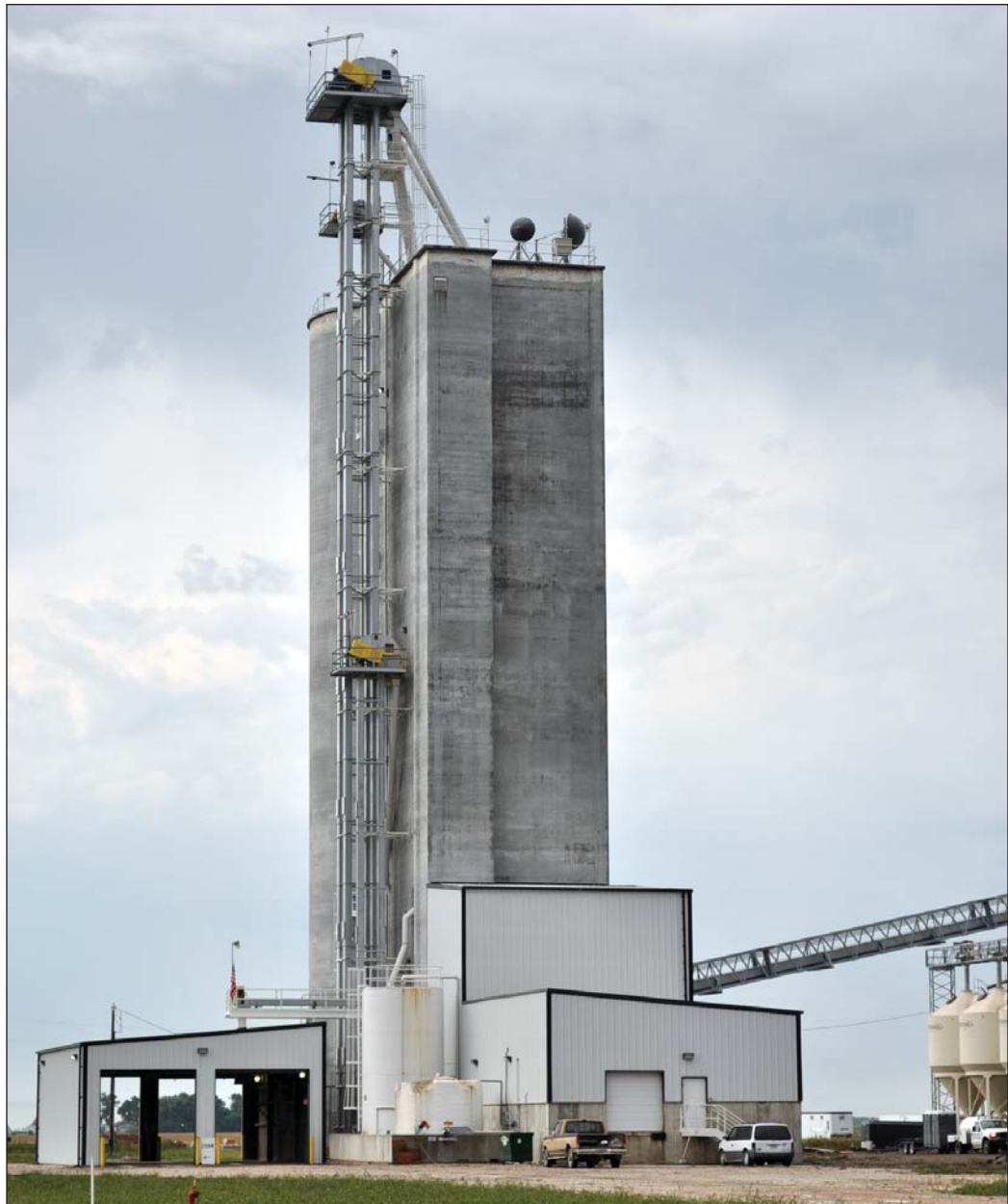
Ground level view of Hawkeye Pride Egg Farms' new 340,000-tpy feed mill located a few miles southeast of Corwith, IA. Photos by Ed Zdrojewski.
