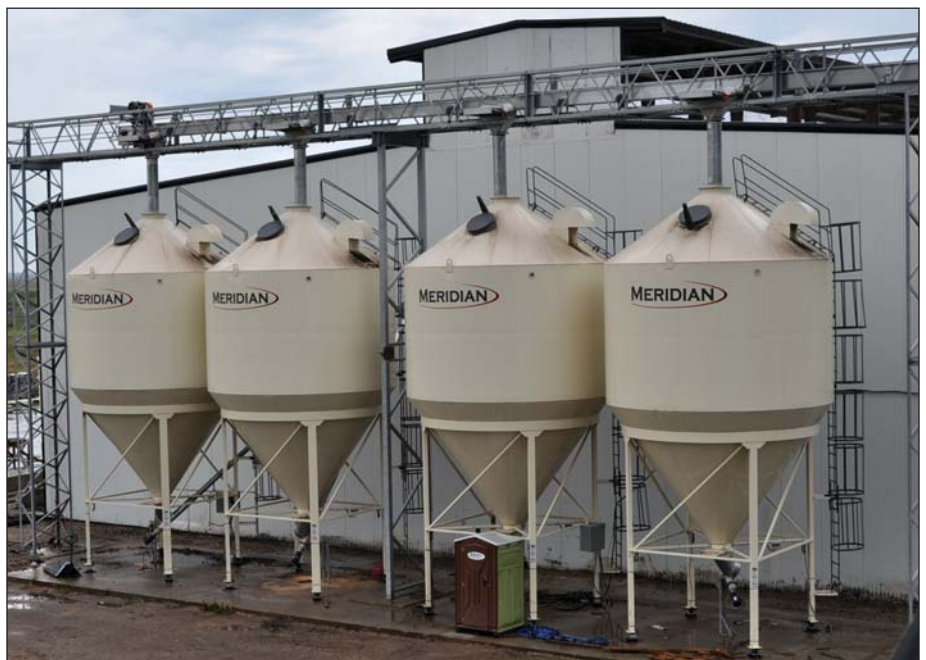
Finished feed is delivered via a series of overhead 5,000-bph Schlagel drag conveyors to storage in 60-ton Meridian tanks serving poultry houses, each containing 680,000 layers.
