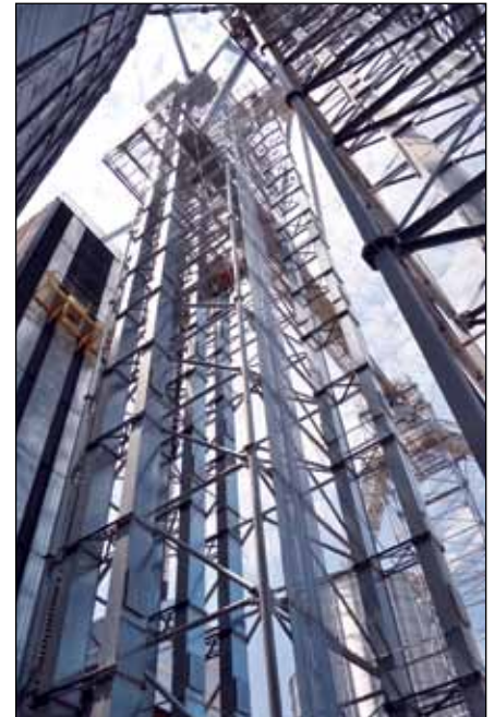
Four 15,000-bph GSI legs, two for receiving plus wet and dry legs for the new dryer, are encased in a Warrior support tower.
