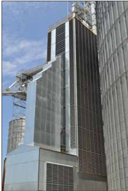
Natural gas-fired, 10,000-bph Shanzer rice dryer is the second rice dryer on the property.
