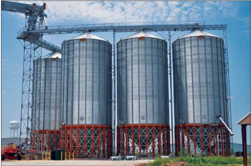
Four of six new 50,000-bushel GSI steel hopper tanks visible provide more separations for both wet and dry rice during and after harvest. Photos by Ed Zdrojewski.
