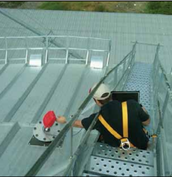
Two 3D Level Scanners provide maximum coverage of the material surface.
