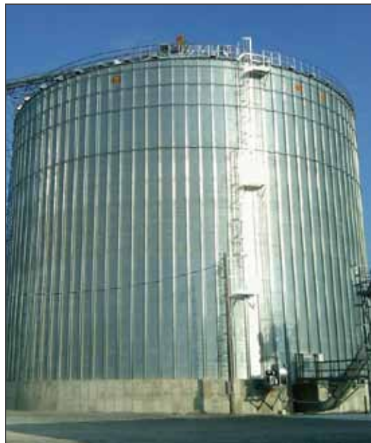
105' diameter and million bushel bins are increasingly popular.
