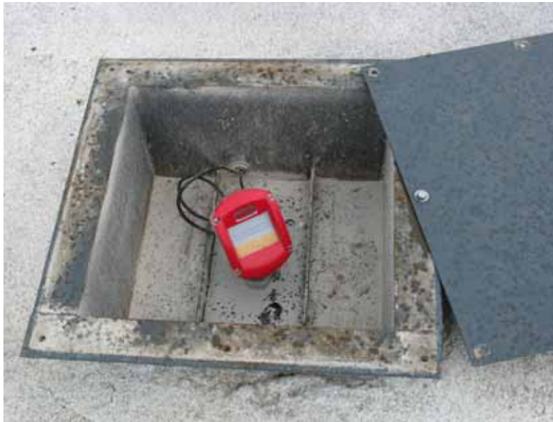
Actual application showing Scanner mounted using existing opening and cover.
