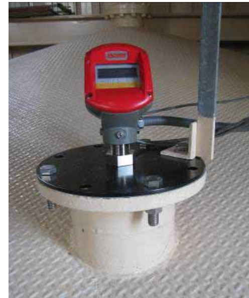
Actual application showing Scanner mounted on existing flange using adapter plate (1/6 in from silo diameter).
