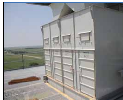
40,000-bph Magik Kleener gravity screener.
