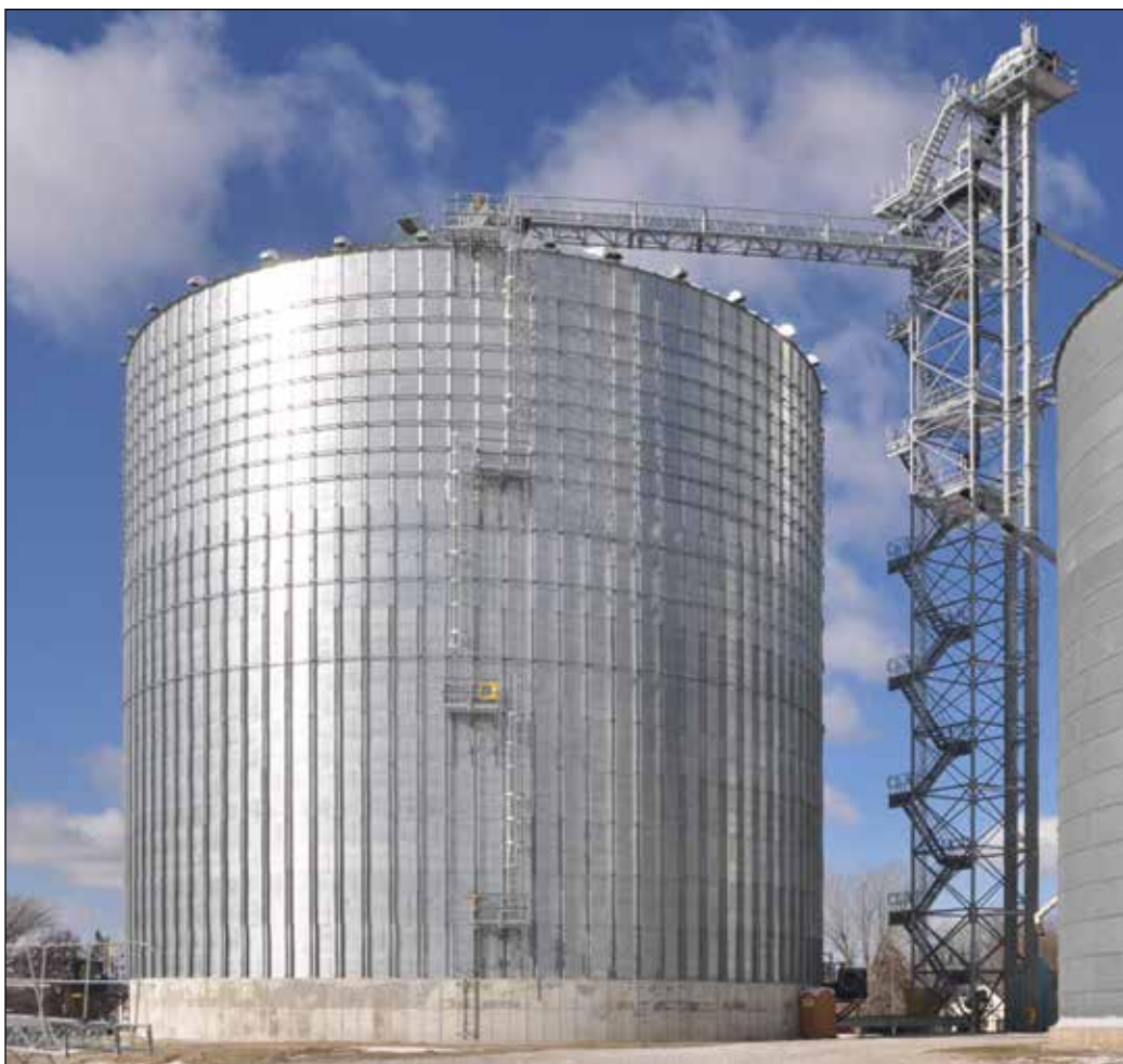
Expansion at Central Valley Ag in Petersburg, NE includes a 750,000-bushel Behlen tank, Schlagel 20,000-bph leg and rotary distributor, and 14-foot-x-14-foot LeMar tower. Photos by Ed Zdrojewski.
