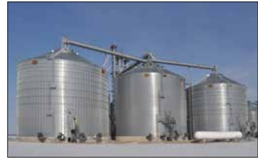
Ground level view of two new GSI 700,000-bushel tanks at far right and left of row. Photos by Ed Zdrojewski.
