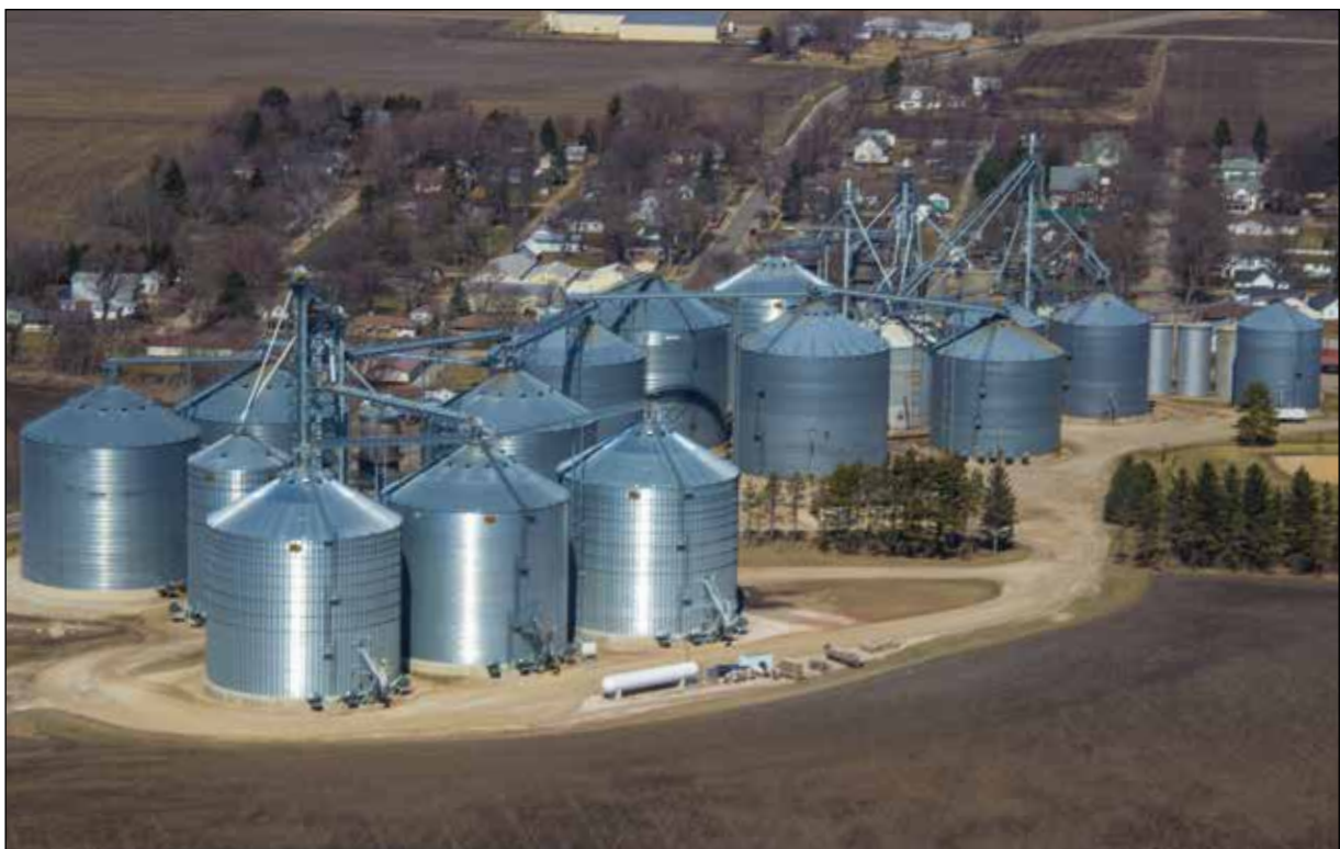
Aerial view of the main Farmers Cooperative Association elevator in Varna, IL, with two new 700,000-bushel tanks bottom center at far right and left of a row of three. Aerial photo by Philip Parker Jr., Urbana, IL.
