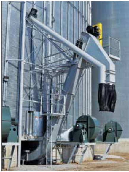
GSI reclaim conveyors end in an incline up to blend grain stream into the sidedraw spout for truck loading.
