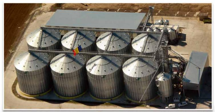
Diameter: 16,81 m - Capacity: 3.395 T - Total capacity: 21.000 T
